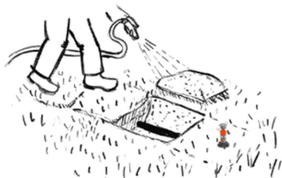
**I** Now replace the soil, lay the turf on the soil and tread down. Everything will grow back faster if you water the soil and turf beforehand. After two to three weeks, you will not be able to see the system any more.
