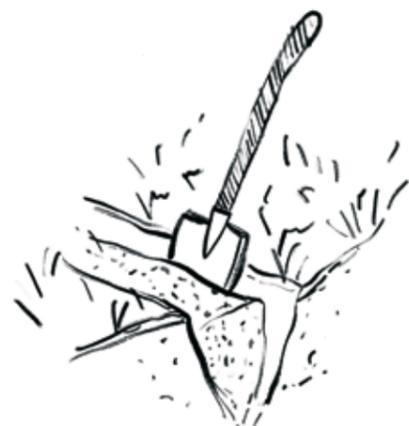
**F** Use a spade to cut out a v-shaped pipe trench approx. 20-25 cm deep. When doing so, carefully remove the turf that you have dug out and dig out the trench. Remove any stones from the trench.
